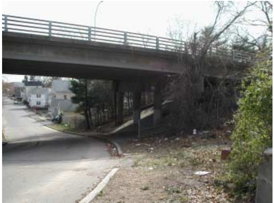
The Smithfield Avenue overpass at Concord Street.
