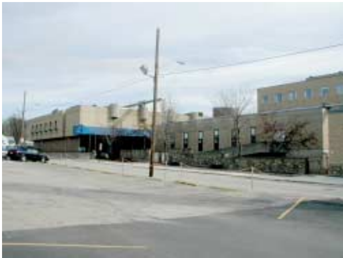
Miriam plans to demolish these two buildings.
