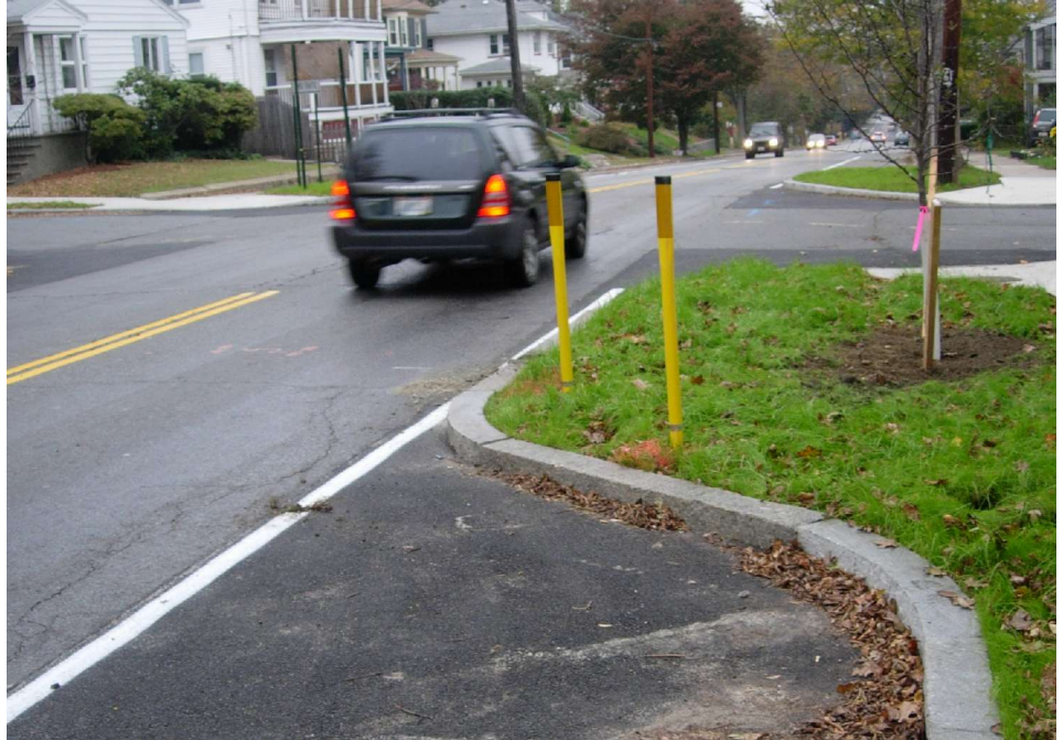
A bump-out at Hope Street and Overhill Road.
