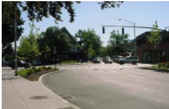
Recent improvements made at Wayland Square
