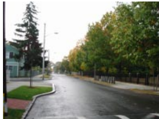
Curb extensions at a Tee intersection in Elmwood.
