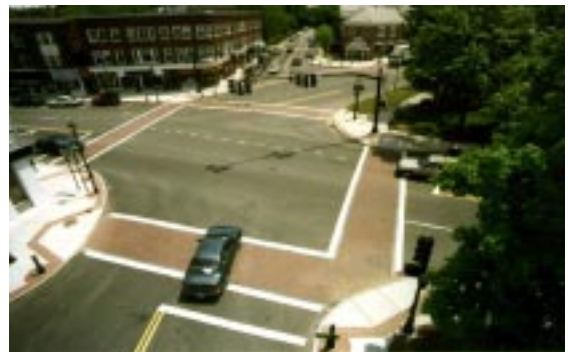
Intersection after improvements.
