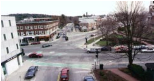
Intersection prior to improvements.
