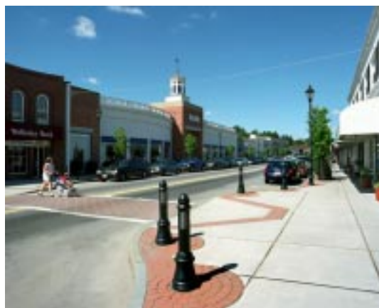
Streetscape improvements including bollards, curb extensions, and brick banding of sidewalks in Wellesley, MA.
